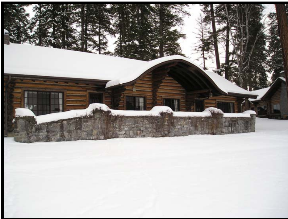
The above photo of the Florman Building, located toward the southern end of the property, shows a stone terrace and curvilinear roof projection that are present on many of the structures.
